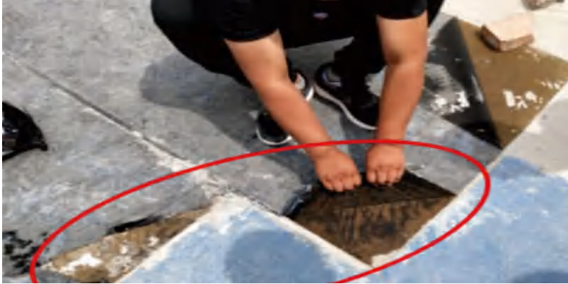
When self - adhesive Waterproofing Membranes are wet - laid, there is no sealing layer.
