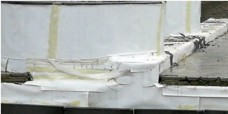
Polymer Waterproofing Membrane materials are stiff, difficult to conform to the surface and hard to seal.
