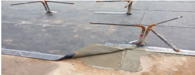
Traditional waterproofing materials fail to address the interface bonding technology. They can't achieve a firm or long - lasting bond, and the adhesion is reversible.
