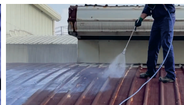
Spraying Special Purpose Interface Treating Agent matched with XINIUPI Protective Membrane 喷涂西牛皮防护膜专用基层处理剂
