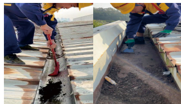
Clean Gutters 清理天沟/檐沟
