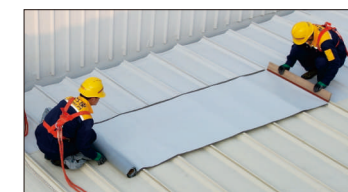
Large-scale pasting/installation 大面铺贴
