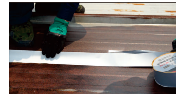
Lap Joint Reinforcement 搭接缝加强
