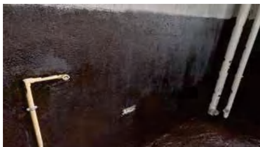
Bathroom Waterproofing 卫生间防水
