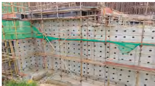
Detailed Waterproofing Treatment for Sidewall Tie-Rods Using Waterproofing Paste 侧墙对拉螺栓使用防水膏细部节点处理
