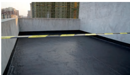
Large-area Waterproofing 屋面大面积防水
