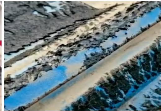
The torching/hot-melt method damages the paint surface of the color steel tile, leading to easy rusting
