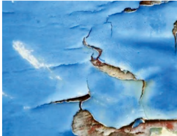
The waterproof coating layer is not resistant to ultraviolet rays and is extremely prone to aging and cracking, with a short service life.
