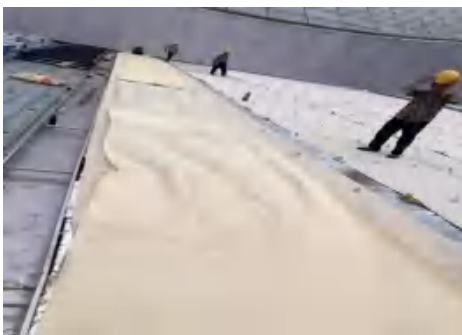
The waterproofing membrane cannot be sealed and bonded with the metal plate, and the air tightness and water tightness of the system are poor.
