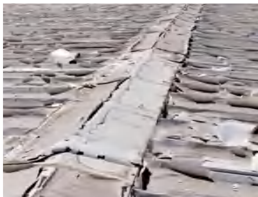
Aging and embrittlement, losing the sealing effect on the nail holes.
