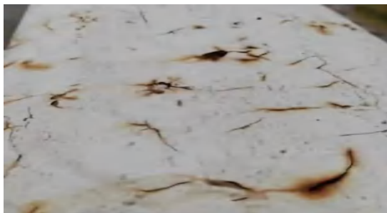
The protective paint film is damaged due to aging caused by metal tremors or acid rain, etc.
