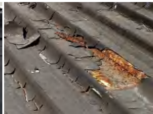
Aging and embrittlement, losing the sealing effect on the nail holes.
