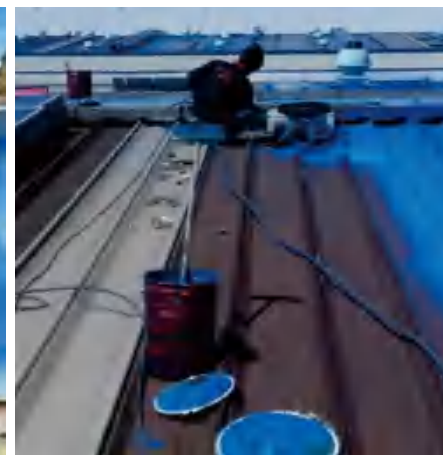
When using the method of manual brushing, it is very difficult to control the thickness of the coating layer, and the situation of cutting corners is likely to occur.
