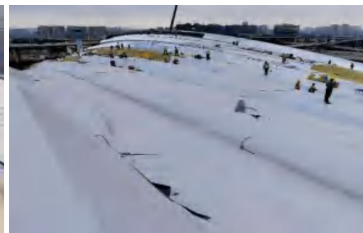
The sheet of PVC waterproofing membrane is stiff, and it is difficult to be fully adhered and sealed on the special-shaped metal roof. Moreover, it is not resistant to aging and large areas of degumming may occur.
