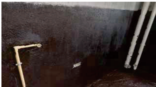
Bathroom Waterproofing 卫生间防水
