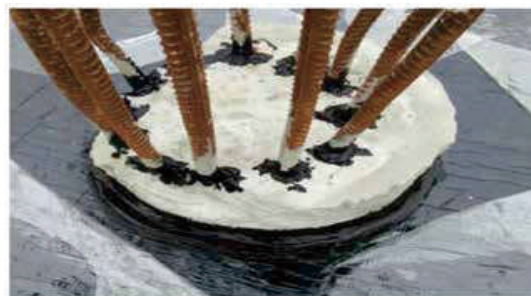
Pile Head Joint Sealing Treatment 桩头节点密封处理
