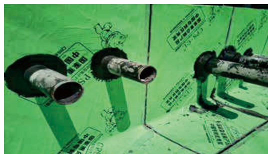
Pipe Penetration Joint Sealing with Waterproofing Paste 管根节点使用防水膏密封处理
